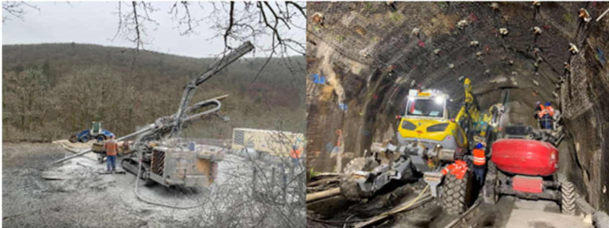
Figure 8. On the left: drilling from above to inject the grout. On the right: drilling from the tunnel for anchoring the deconsolidated soil injected above the hole in the vault
