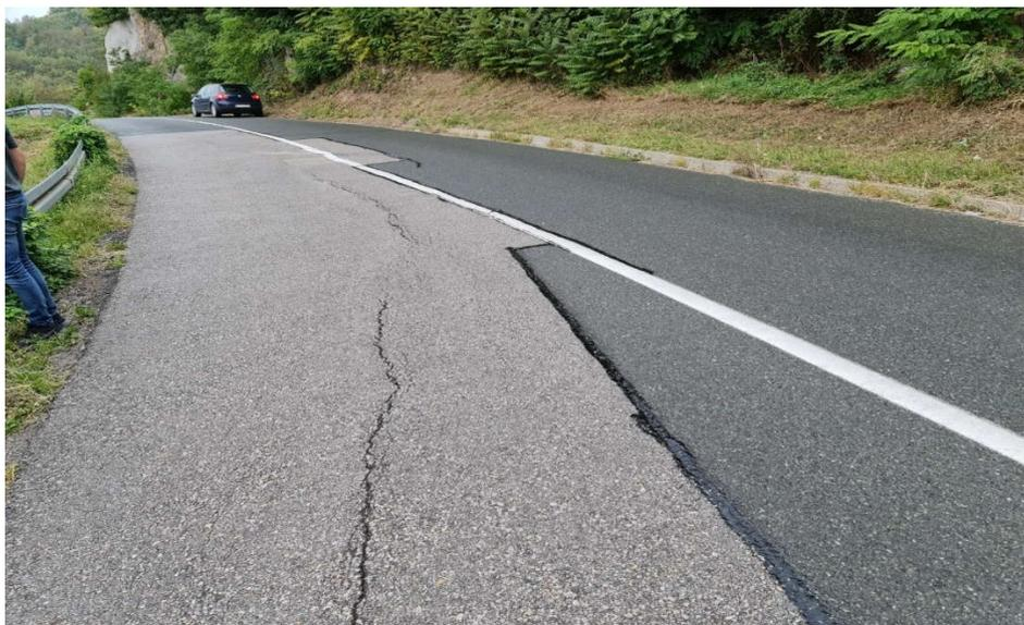
**Figure 17.** Western part of the road with developed crack about 15 meters long
